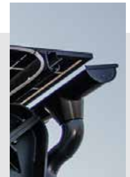
Gutters and sheet metal roof
