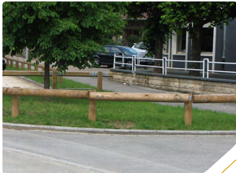
Tonçons courts - Parking
